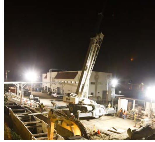
Influent pipe installation – Encina
